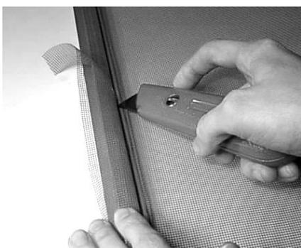
Note: When trimming mesh use the knife at angle *shown below*.
