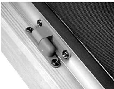
**14.** Fit the turnbuttons with a single screw to the window frame, so when pivoted they overlap onto the lip of the flyscreen profile.
